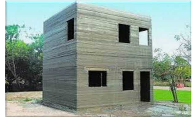
L&T printed a G+1 using Gantry at Kanceepuram - 2021
