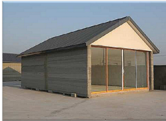
House printed by Win Sun company in China - 2014
